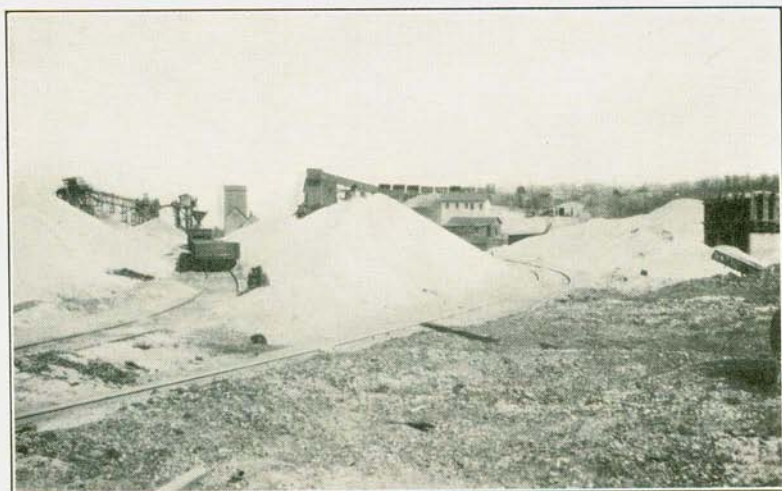
(a) Bennet plant of the New Jersey Sand and Gravel Company, located three miles east of Farmingdale, Monmouth County.
