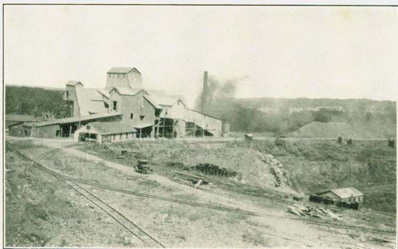
(a) Plant of the Morris County Crushed Stone Company (trap rock) at Millington, Morris County.
