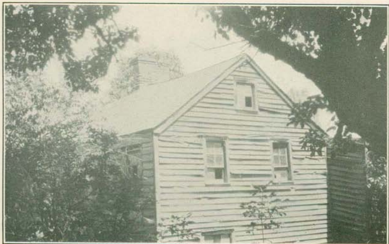
(b) Sixty-year-old house in Lafayette roofed with slate from the Lafayette quarry. The slate is still in perfect condition.
