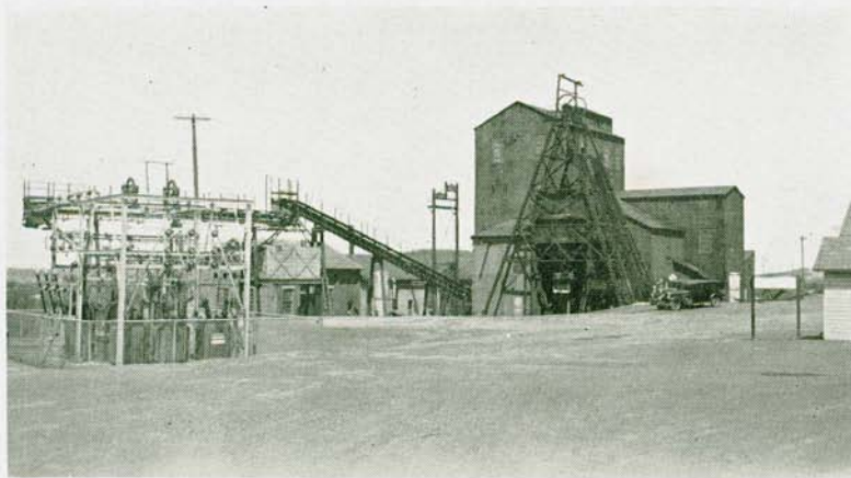
A. Headframe, mill, loading conveyors and electrical transformers at the Washington Mine of the Alan Wood Mining Company near Oxford.
