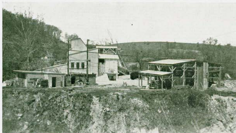
B. Crushing plant at the Lizzie Clay Quarry of the Jersey Materials Company, situated north of Phillipsburg. NEW JERSEY GEOLOGICAL SURVEY
