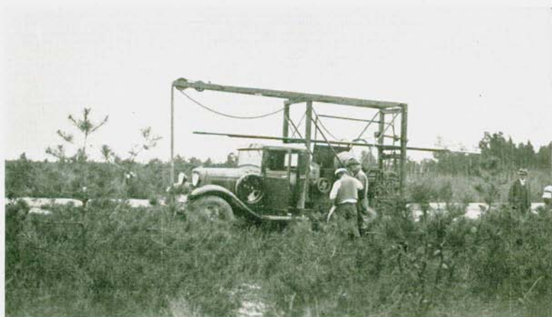
B. Light and compact, hydraulic drilling rig used by the U. S. Geological Survey for drilling test holes in sandy terrain
