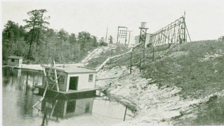
A. Dredge and part of the "silica sand" plant constructed by the Peerless Sand Company in 1935 and situated two miles north of Lakewood.
