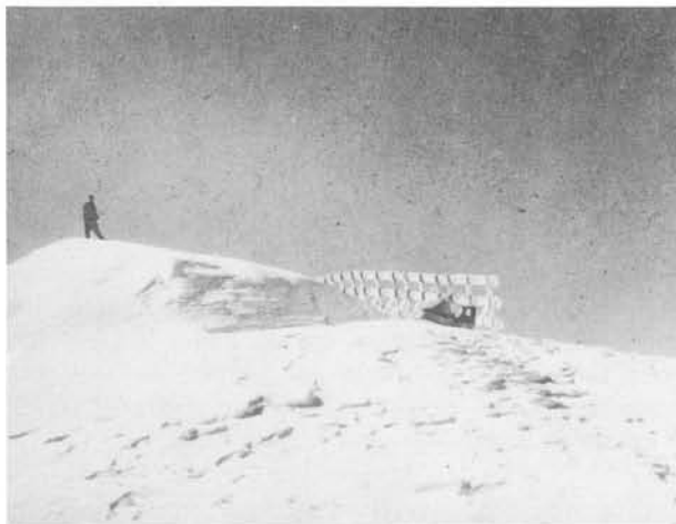
Figure 2. Snow fence on continental divide, note induced drift.
