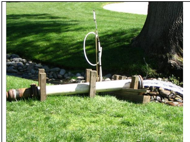
Figure 7. Arrangement of orifice weir and vertical piezometer tube for measuring discharge of pumping well. (Photo by S. W. Johnson.)
