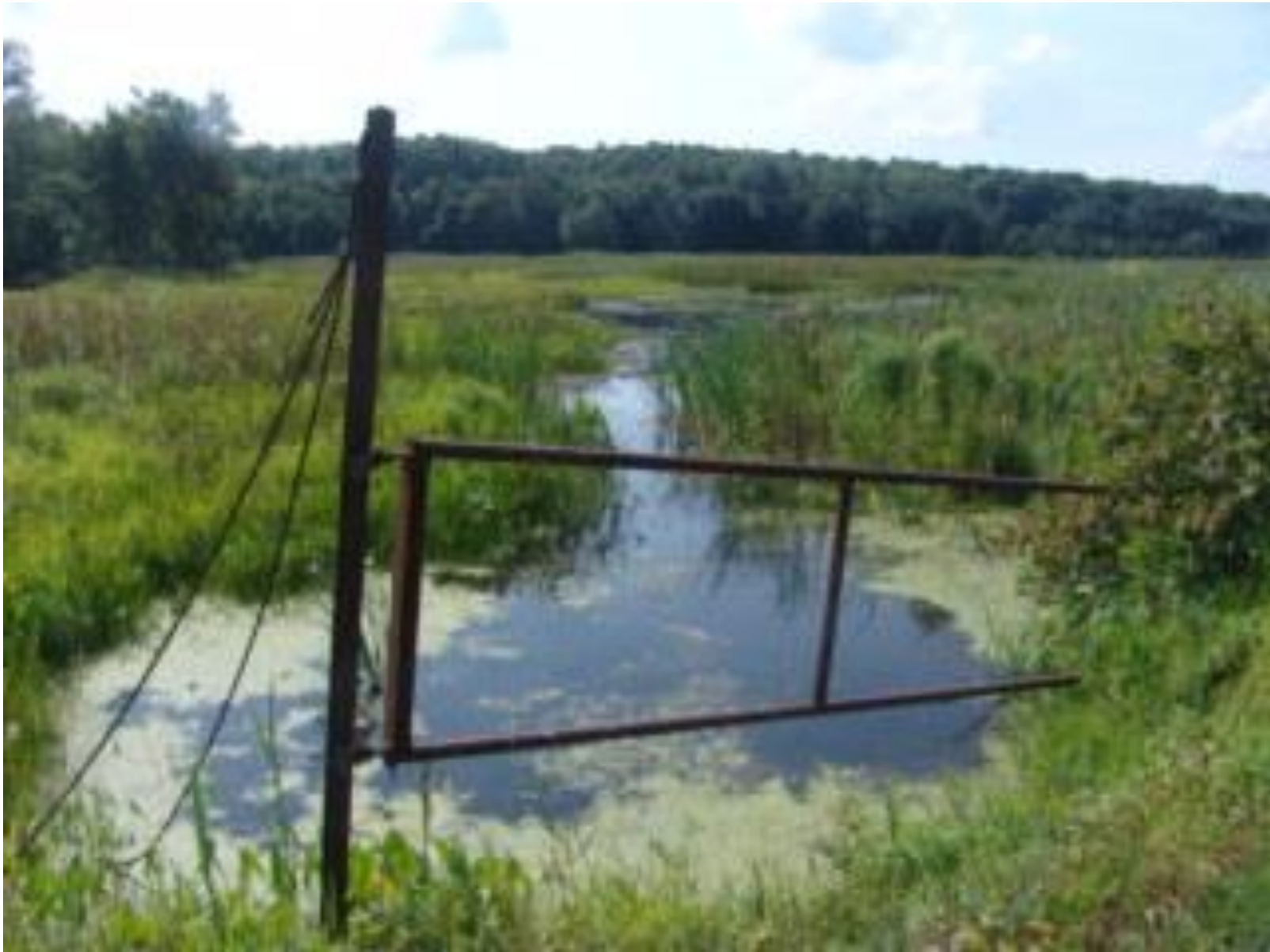
Photo point 2: Looking east at site of water control structure replacement
