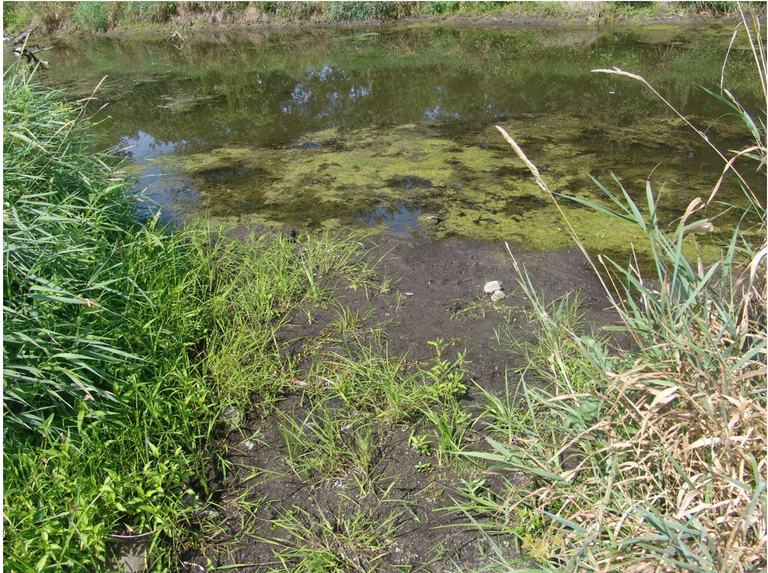
Photo point 5: Existing breach to be repaired
