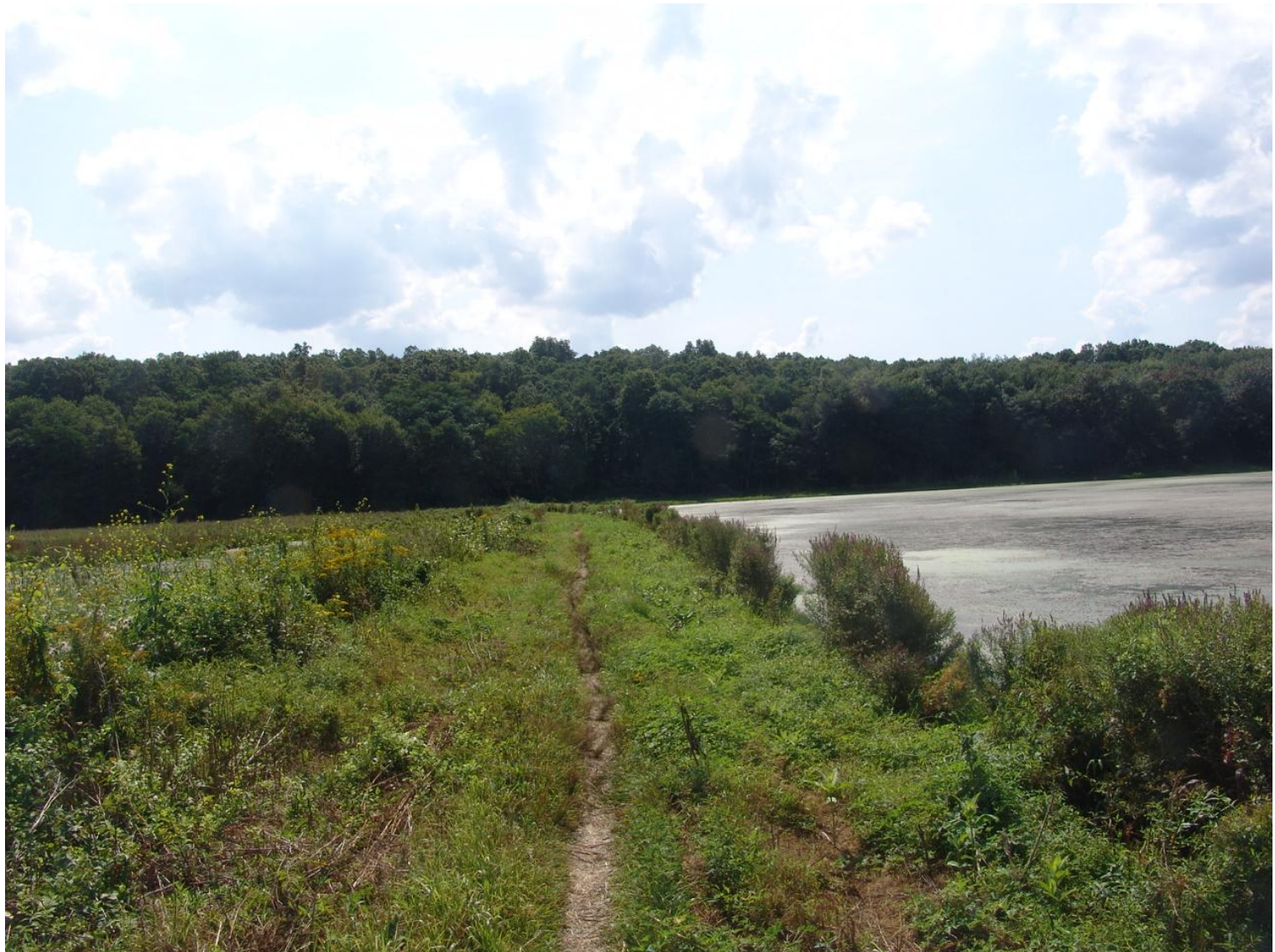
Photo point 4: Looking east along berm
