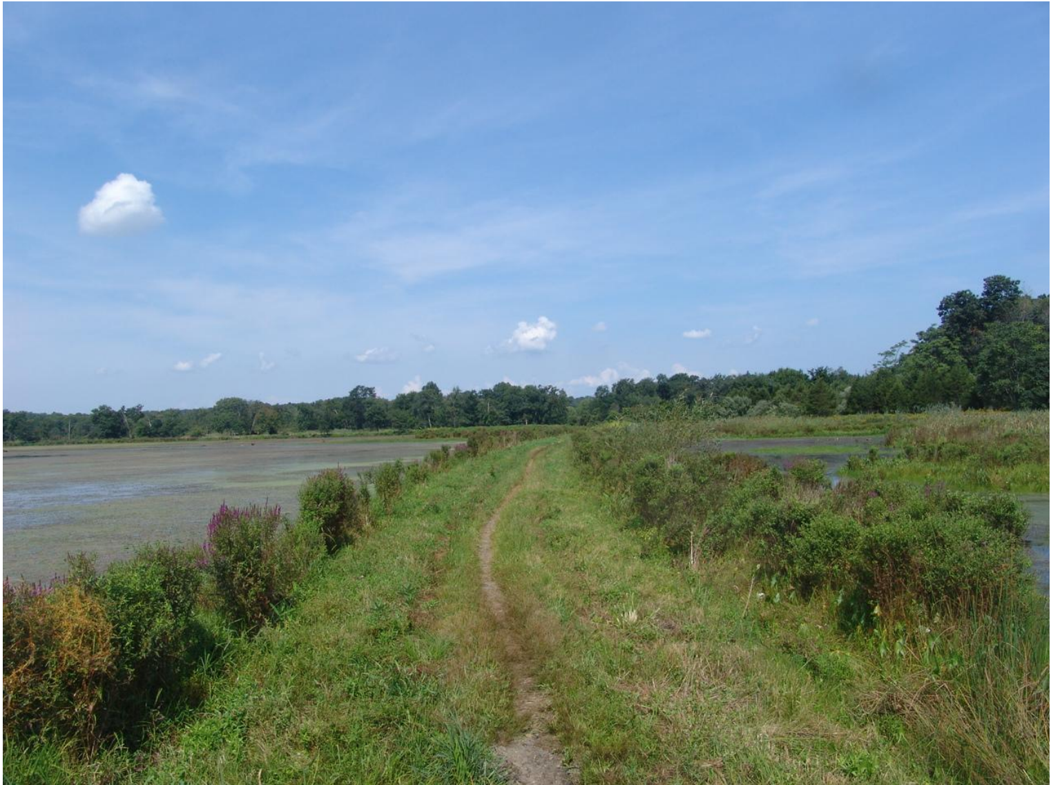
Photo point 4: Looking west along berm
