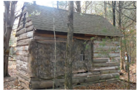
"Thoreau" cabin built by PLC students
