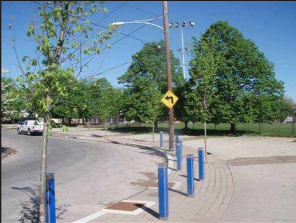
Permeable Pavers, Subsurface Infiltration, Disconnected Inlets
