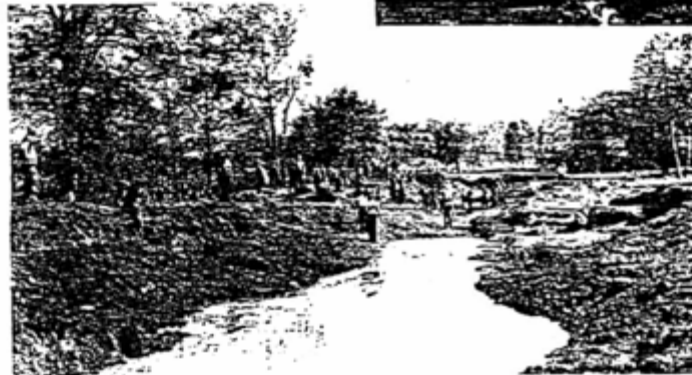
Immediately after explosion, water is entering new channel, whose banks will be smoothed and "stream-lined" by the speedier flow of water.
