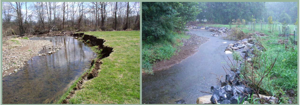
Fig. 8.2. Example of enhancement: Streambank erosion on Walnut Brook. Left April 2007, Right August 2009
