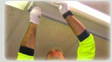
A contractor installs efficient, electronic T5 lights.
