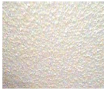
Trowelled on asbestos
