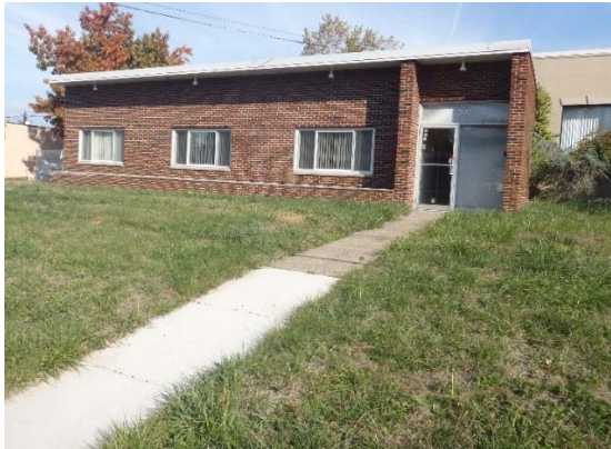
Front of Unimatic Site Building
