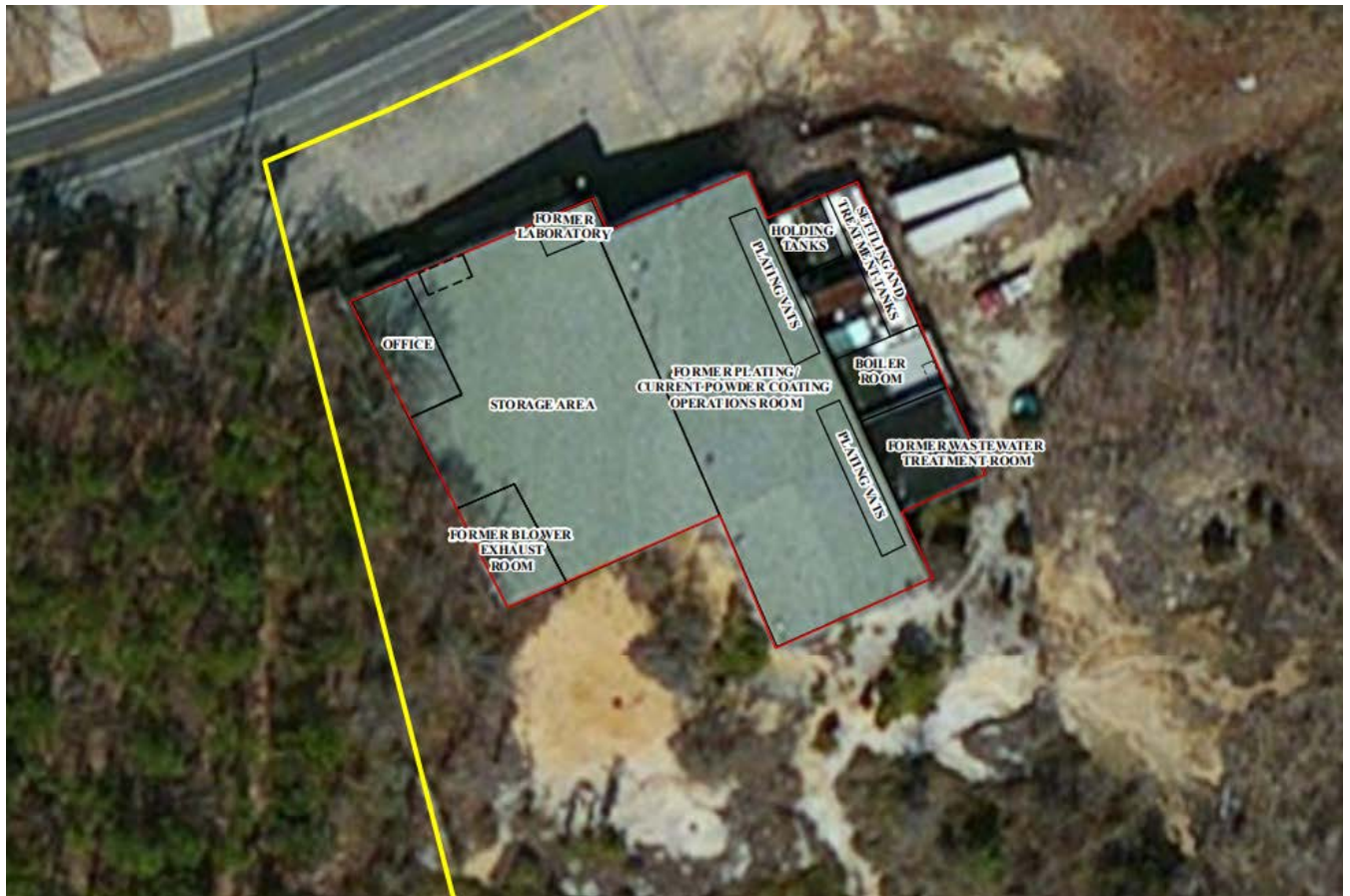
Figure 2. Pioneer Metal Finishing site building
