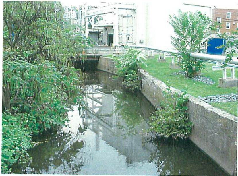
Mile Run Brook on Rhodia Inc. site.
