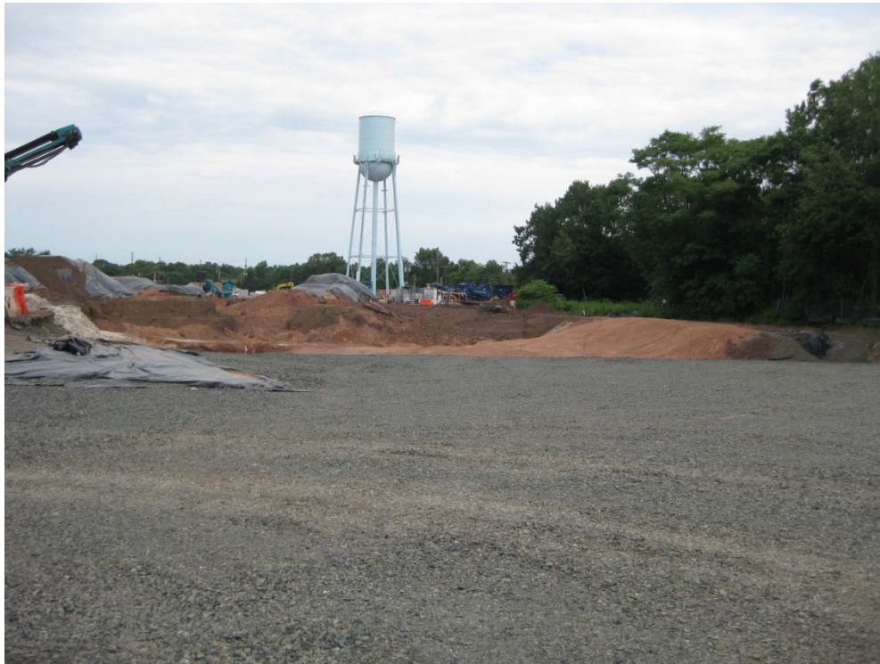
Photograph 3: Construction of storm water detention basin at southeast area of site.
