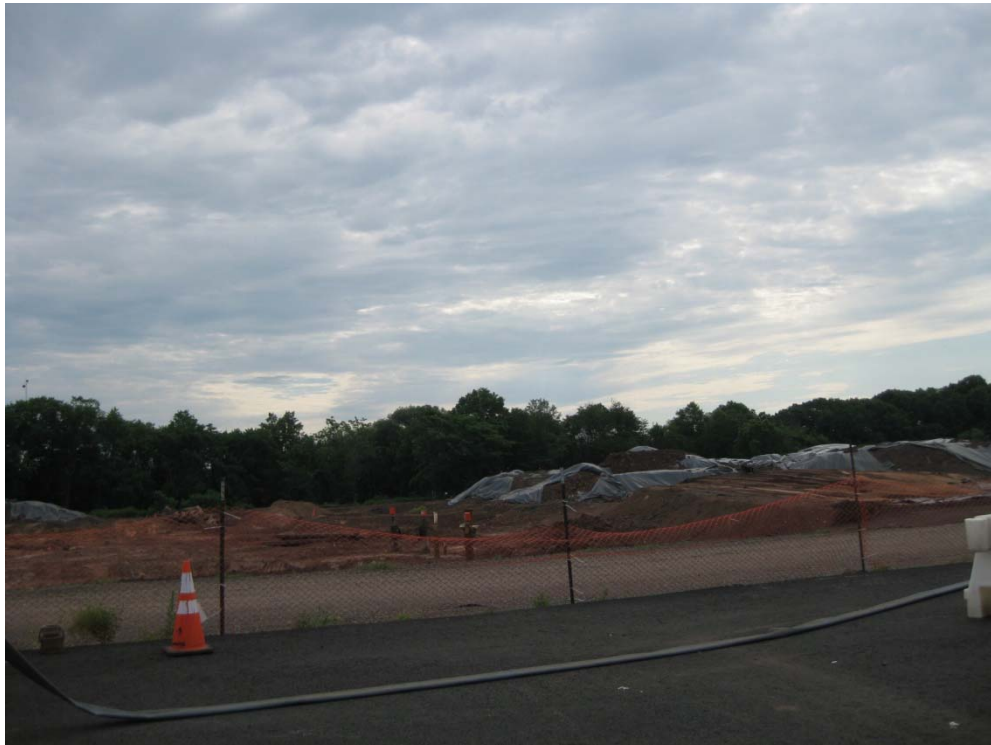
Photograph 2: Soil remediation activities along the northeast portion of the CDE property.
