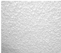
Trowelled on asbestos
