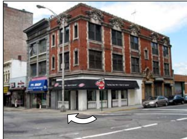
Photo 2 Incident Site Arrow indicates direction of turn
