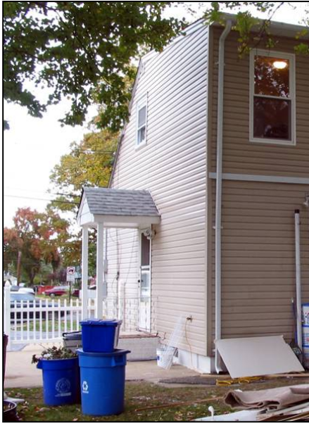
Photo 2 Porch roof peak used to support the scaffold plank
