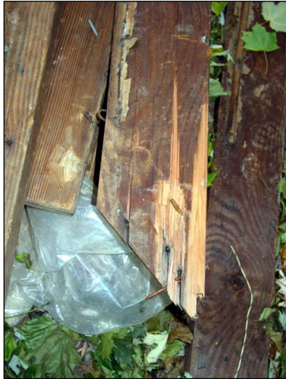
Photo 1 Damaged wood used to make the improvised scaffold
