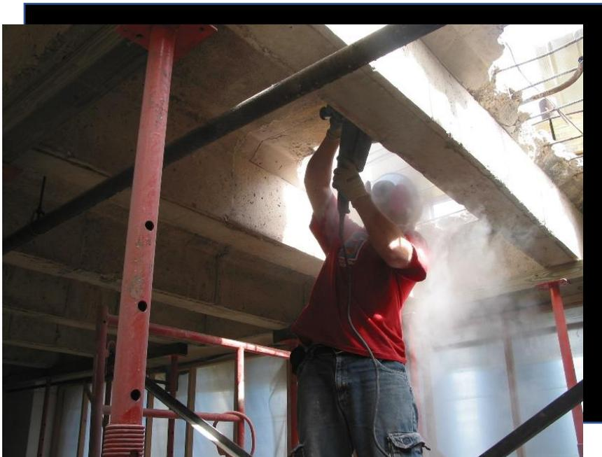
Construction worker exposure to silica dust while cutting concrete during parking garage repair
