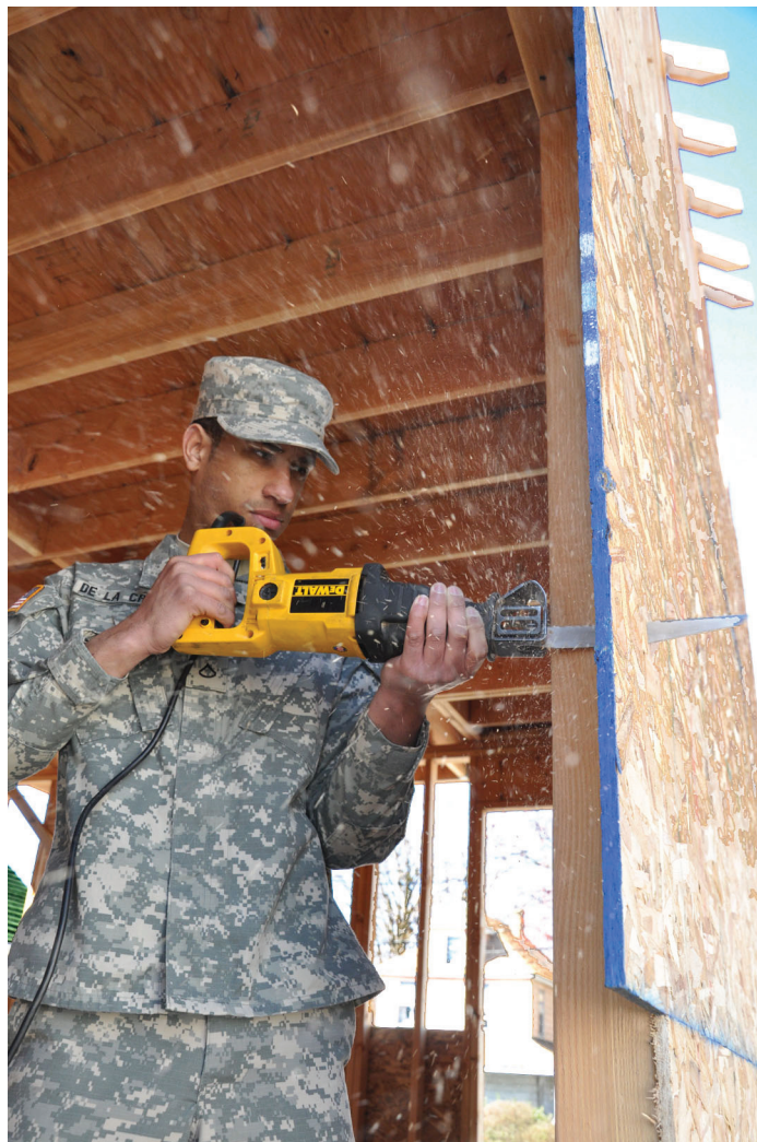
Sawdust flies as Pfc. Hector De La Cruz cuts out a window with a reciprocating saw while on assignment with the Recruit Sustain Program at a Habitat for Humanity project in Asbury Park on March 19. Photo by Kryn P. Westhoven, DMAVA/PA
