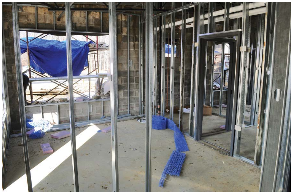
The Public Information Center office wall structure is defined with the addition of studs, sill plates and door openings. (New Jersey Department of Military and Veterans Affairs photos by Kryn P. Westhoven/Released)
