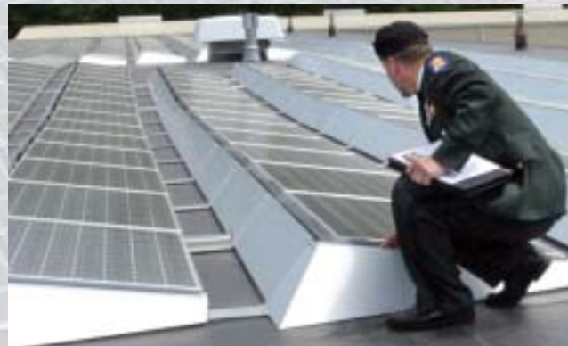
Maj. Erik Myhre, Facilities Manager, checks a solar panel located on the roof of the Homeland Security Center for Excellence in Lawrenceville.
