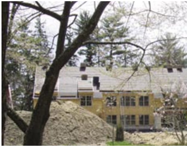
Georgian Court University: Residence Hall
