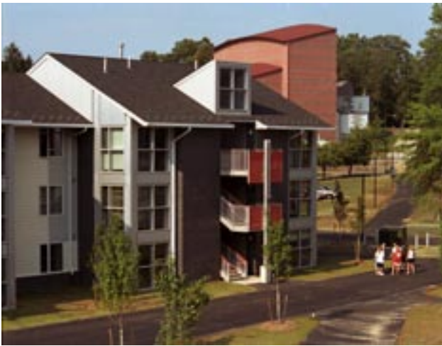
Ramapo College: Phase VII Apartment Residence
