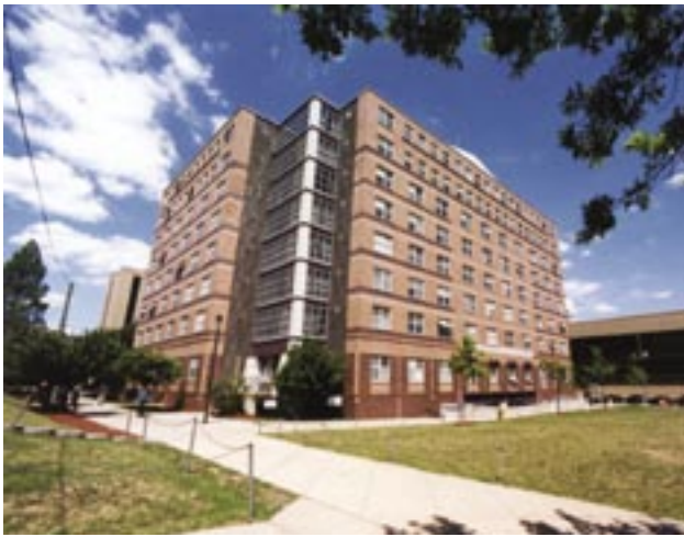
New Jersey Institute of Technology: Cypress Hall
