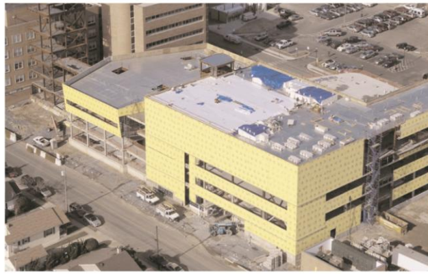
Construction site – February 2010
