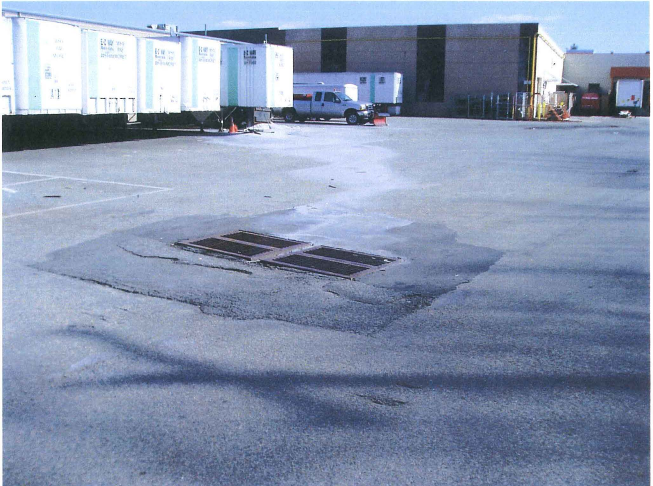
Figure 14 - Careless salt storage flows off the pavement and directly into the nearest waterway. Who's watching after approved site plans are put away and archived.
