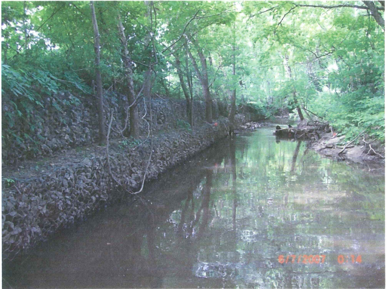
Figure 5 - Eventually even more drastic structural stream bank replacement becomes necessary - Beaver Dam Brook.
