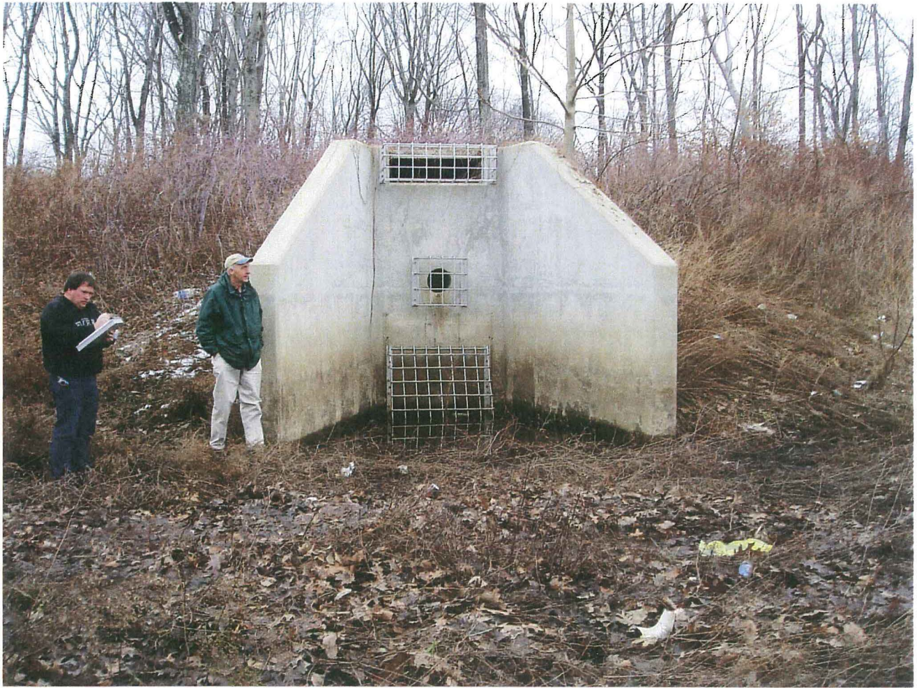
Figure 8 - The installation of storm water retention and detention basins was supposed to ameliorate the peak flows of storm water runoff from each development site. No one has looked to see if such unsynchronized discharges are additive, thereby producing the damaged stream corridors seen in Figures 1 through 7.
