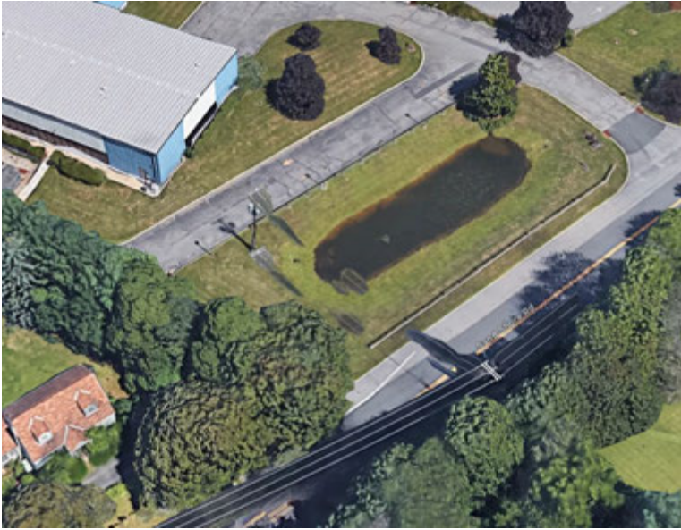
Block 8300, Lot 9 Retention Pond
