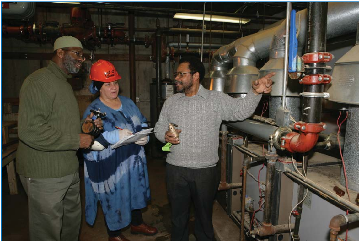
Parolees participate in the boiler room training in order to receive their "Black Seal" certification upon completion of the program.
