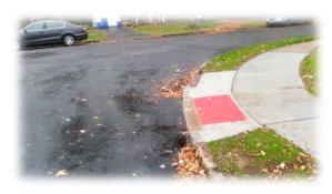
roadways. IH is also responsible for construction management services and community involvement. The project is in construction closeout. The project photo shows one of the newly installed ADA ramps immediately adjacent to a reconstructed drainage inlet. This location previously had a non-ADA compliant ramp with a ponding issue.
