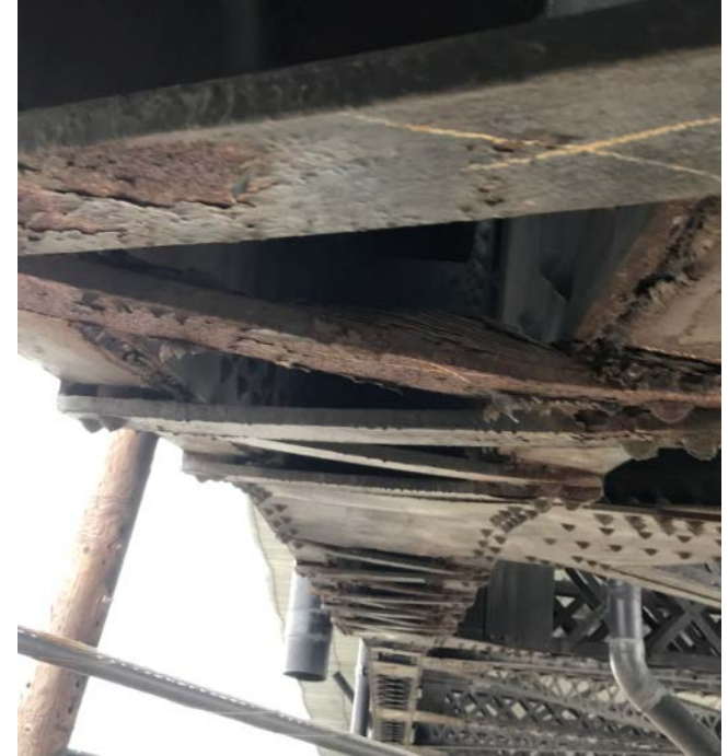
Span 47 Lacing Bars
