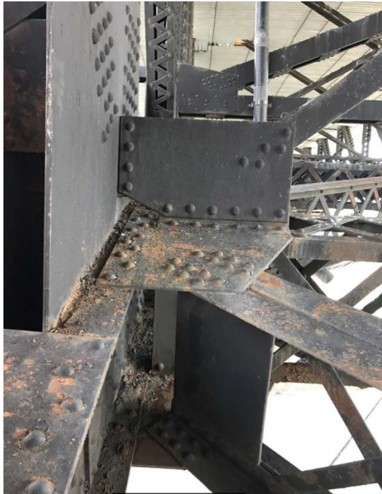
RB47 Bottom Connection Corrosion
