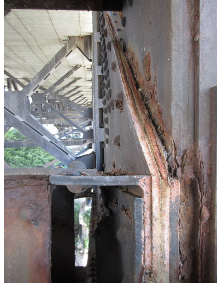
Corroded Slip Surface
