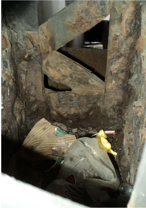
RB47 Vertical Chord Corrosion
