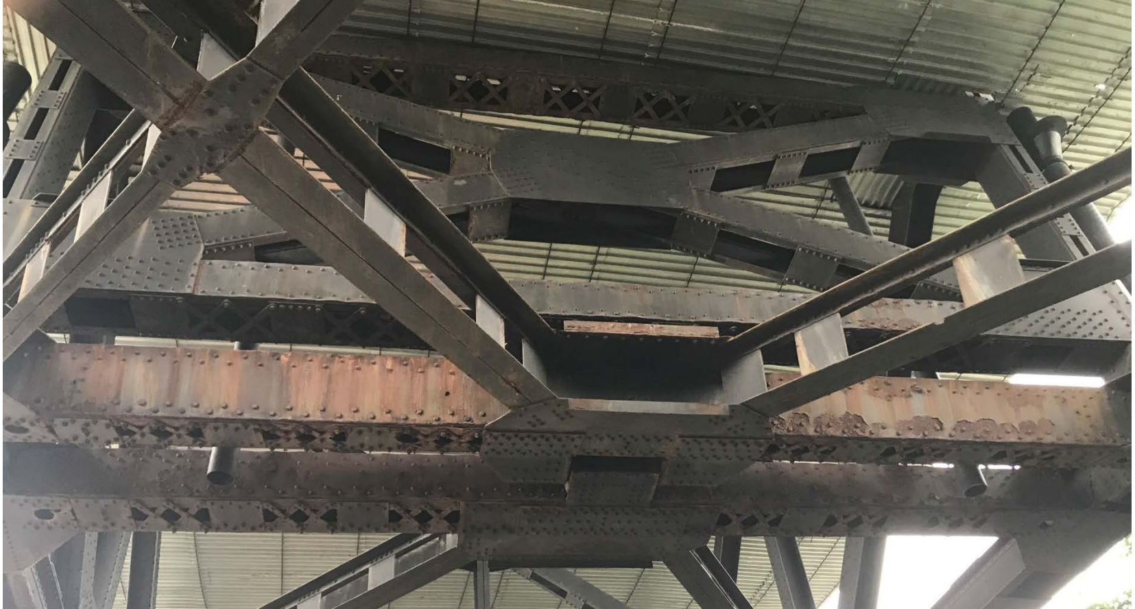
Widespread Corrosion
