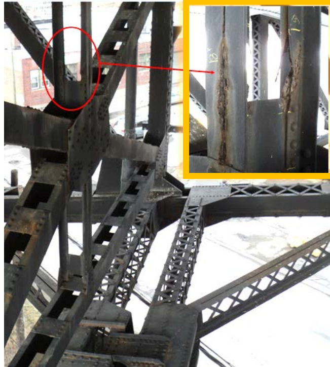
RB47 Sway Brace with Severe Section Loss
