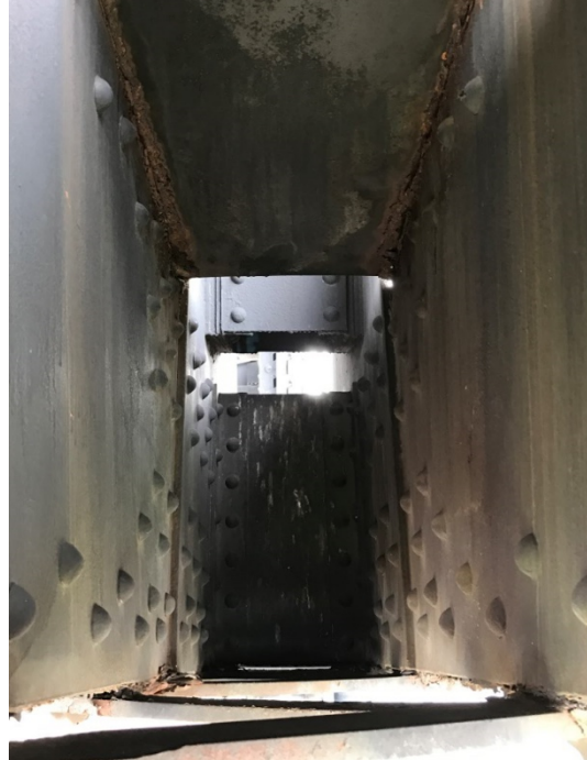
Span 47 Bottom Chord Pack Rust
