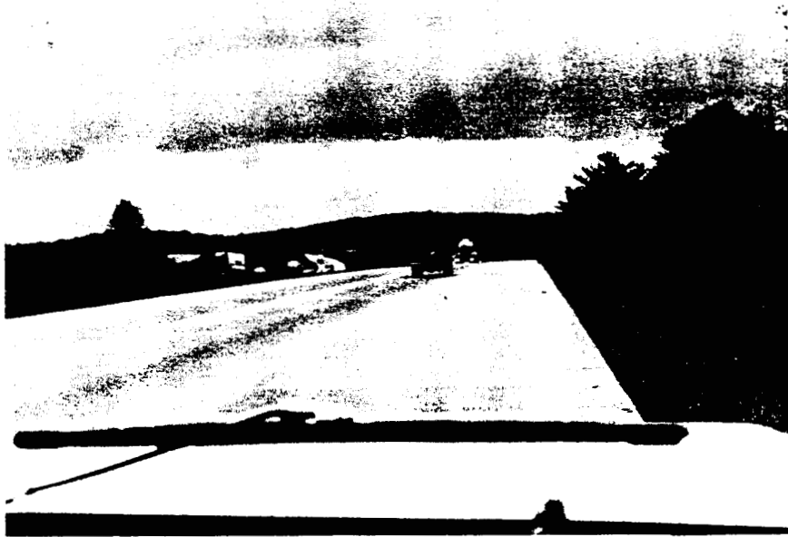
Figure 4. Overview of tied portland cement concrete shoulder section
