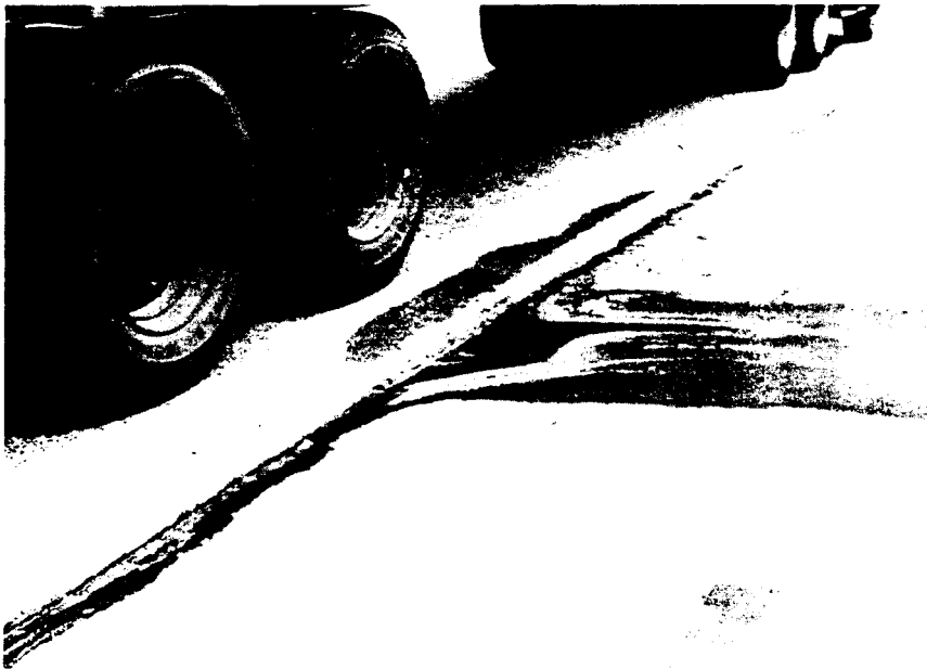
Figure 11. Pumping slabs in LFA inlay section
