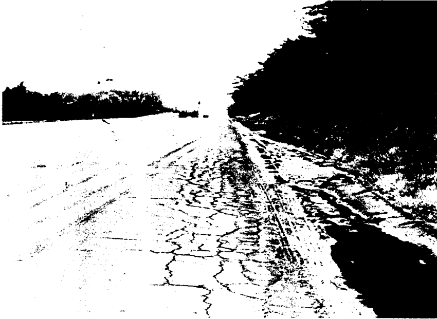
Figure 14. Alligator cracking in I-4 inlay section (Note standing water in truck pull-off area at shoulder edge.)
