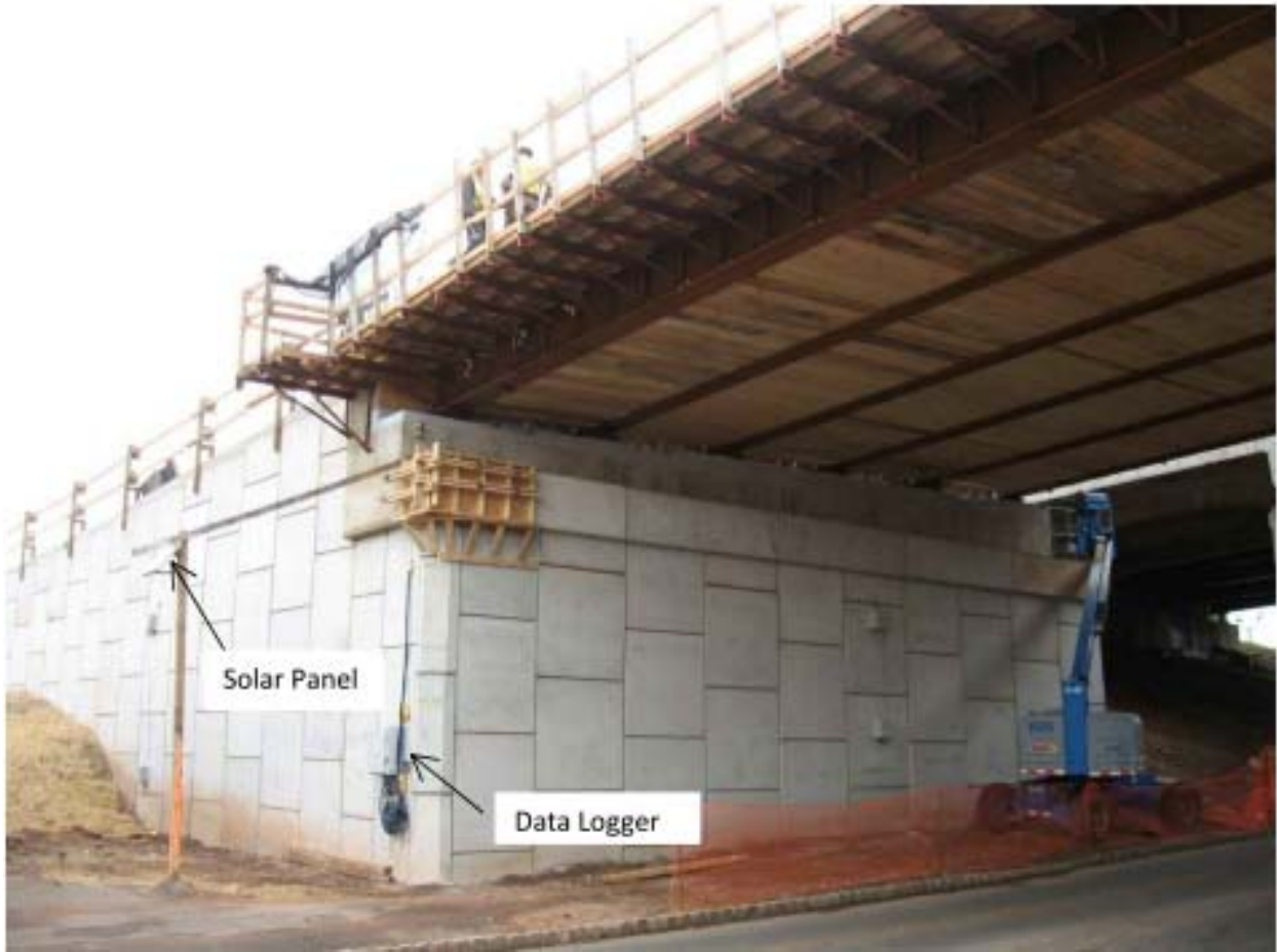
Figure 23. Wall 1 and Wall 3 at End of Construction
