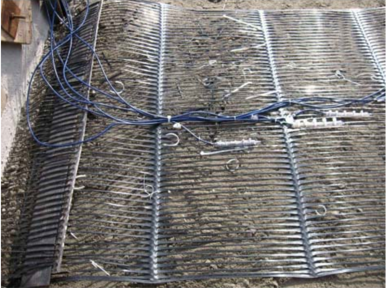
Figure 21. Instrumented Geogrid with Strain Gages
