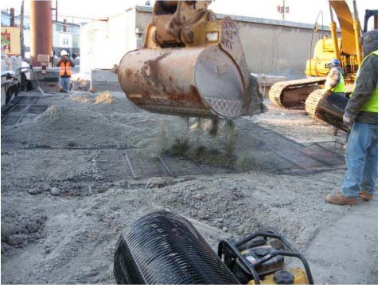
Figure 22. Place Select Fill on Top of Geogrid
