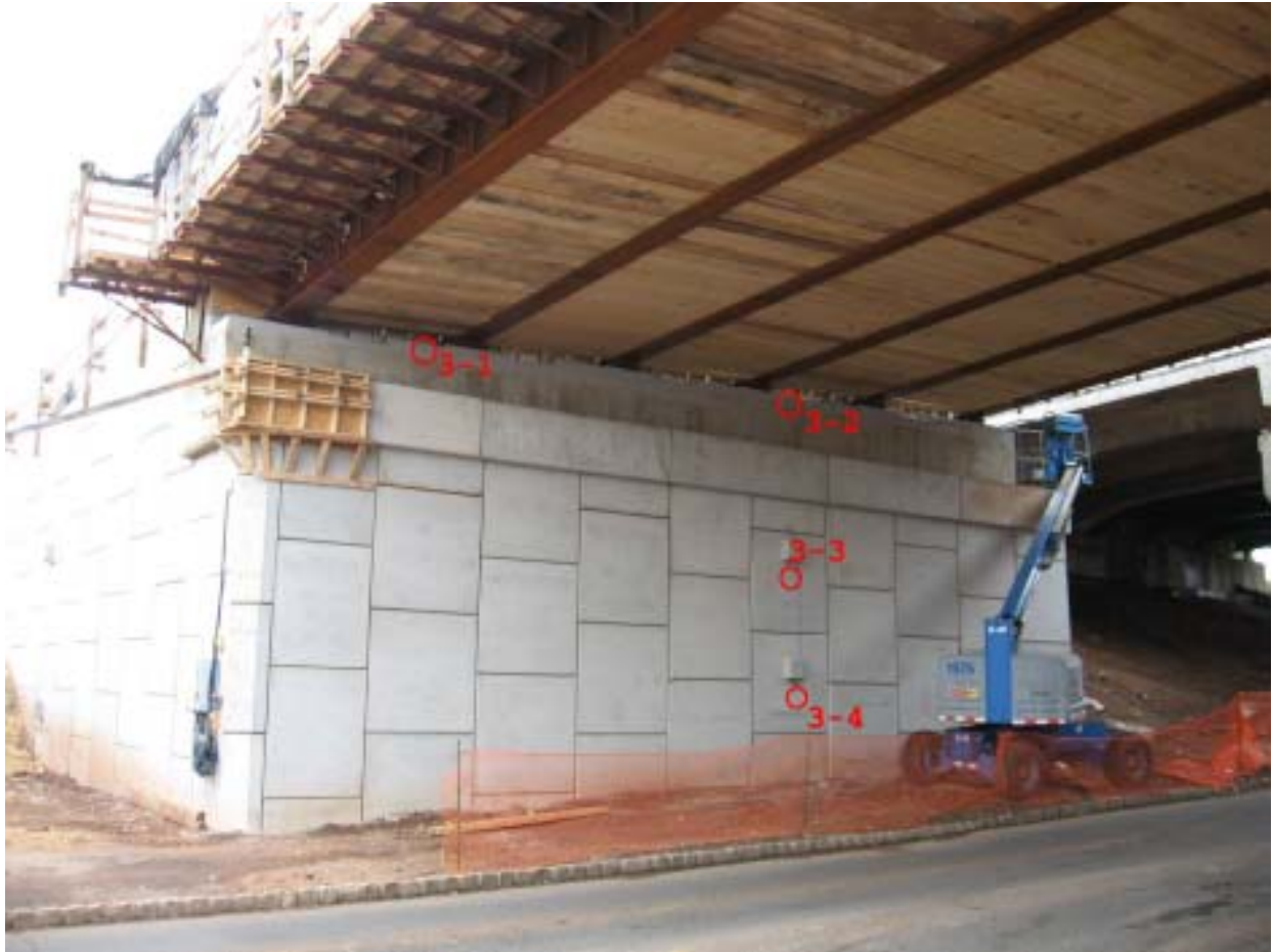
Figure 36. Wall 3 Survey Point Locations
