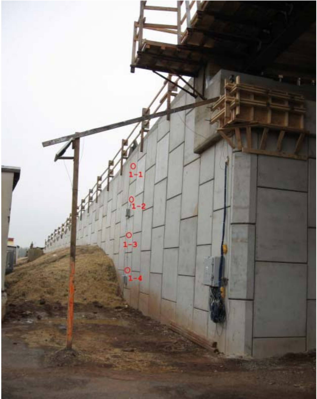
Figure 35. Wall 1 Survey Point Locations
