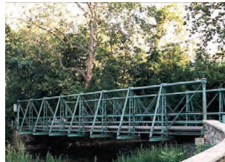
Pony Pratt Truss Bridge Copyright P.S. Green
