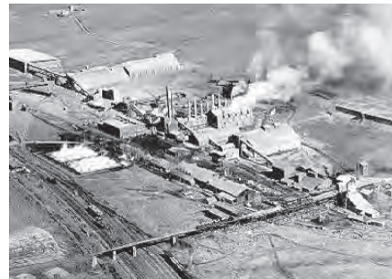
View of Former Edison Portland Cement Company
