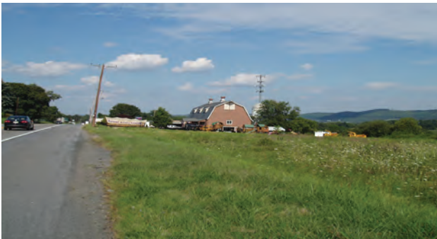
Cell tower at Sunshine Tree and Landscape
