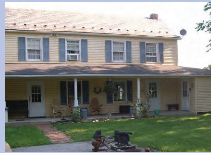
Lift Keeper's House and Excavated Materials
