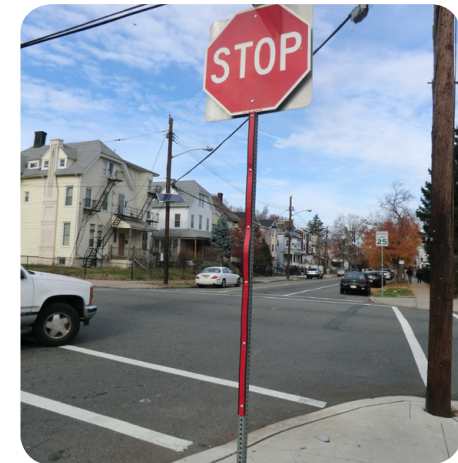
Reflective tape on stop sign post in Newark, NJ. Image: The RBA Group
