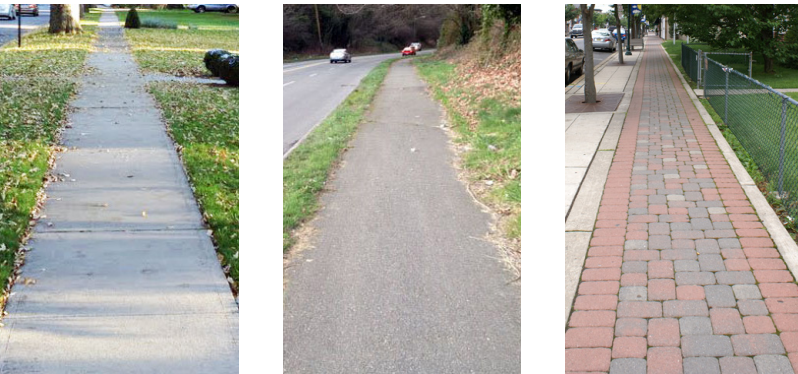
Examples of concrete, asphalt and brick paver sidewalks.
