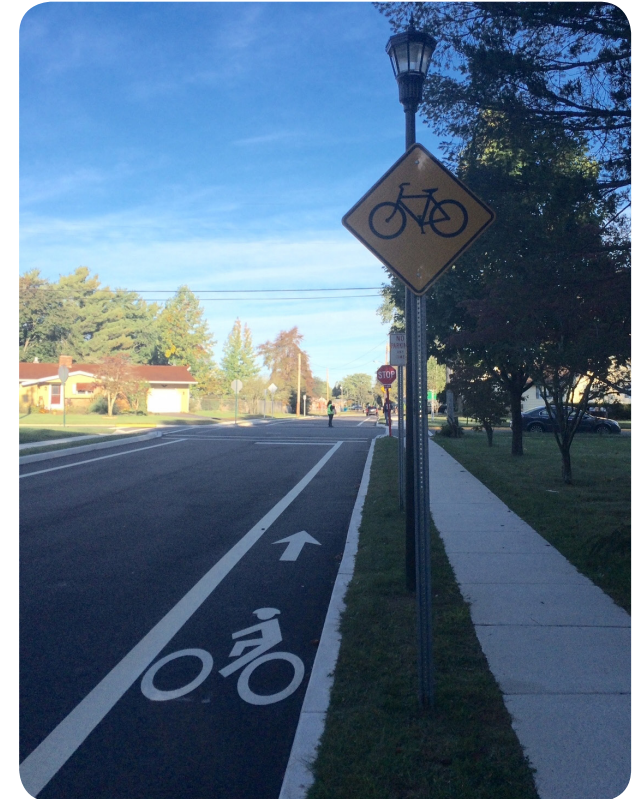
A newly striped bicycle lane on Diesterweg Street in Egg Harbor. Image: NJDOT
