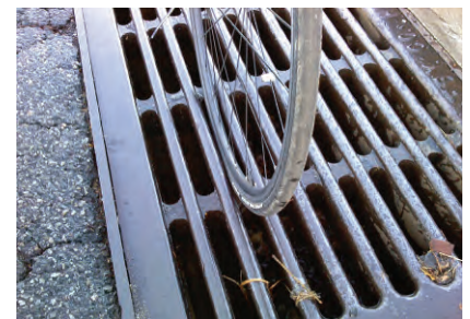
Stream Flow Grate
