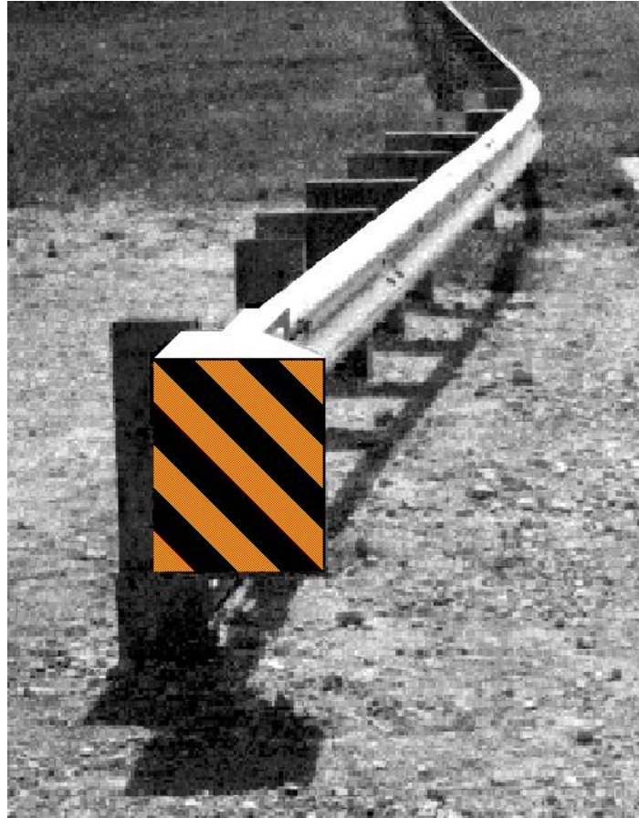
FLARED ENERGY ABSORBING TERMINAL (FEAT)
