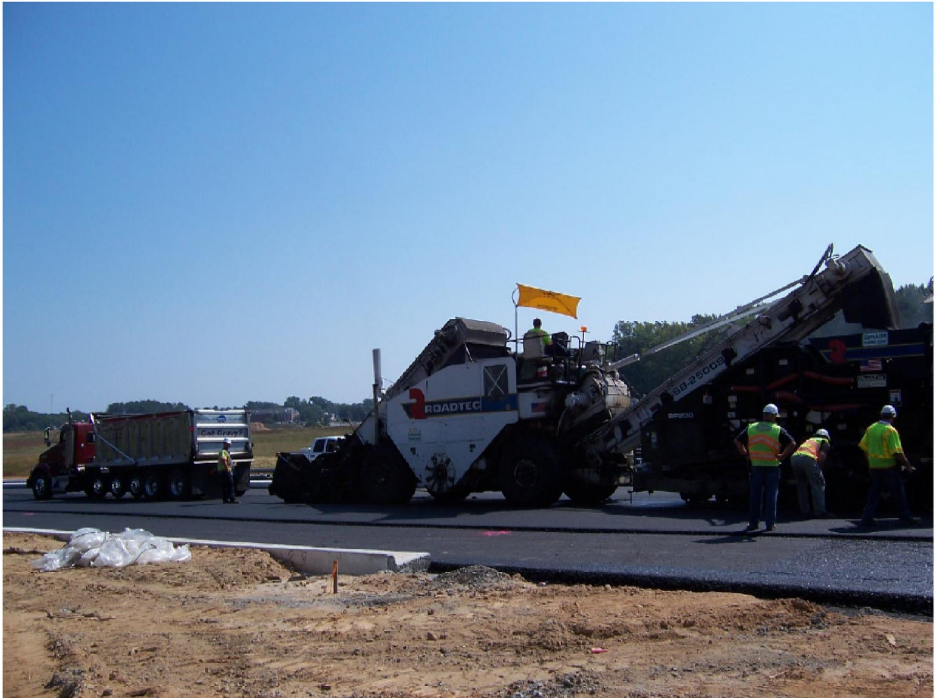
**Except for the weight of the paver screed, the remaining density is achieved through rollers**
