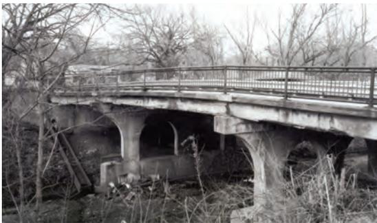
*Route 27 (Lake Avenue) Bridge over LVRR, Metuchen, New Jersey in 2007 (Source: RGA files). This concrete-encased steel stringer bridge was the preferred bridge type of the State Highway Department between the two world wars.*
