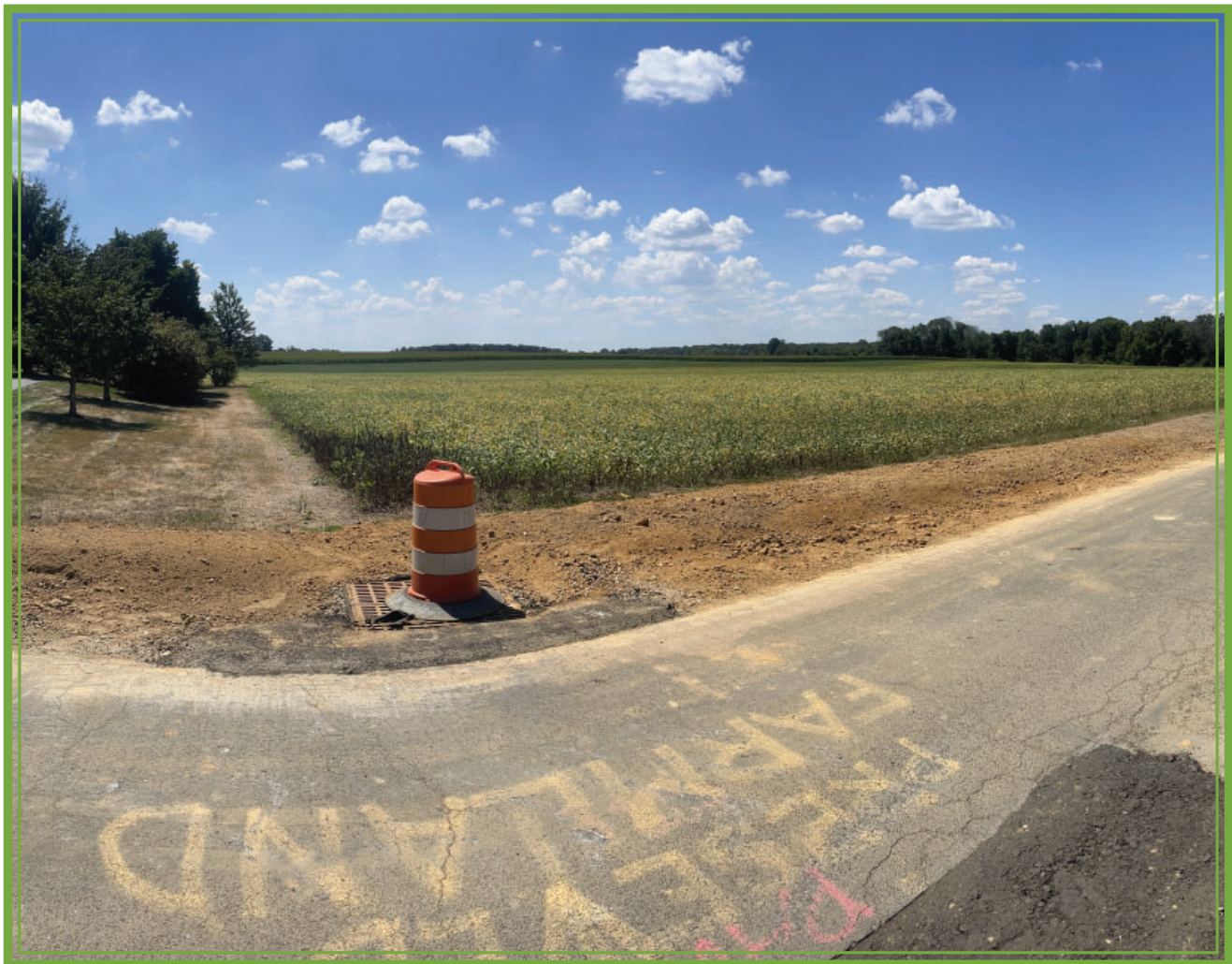
Sewer Line, Middlesex County, Photo by Steve Bruder
