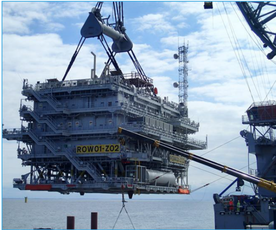
Figure 2-26. Installation of an offshore substation.
