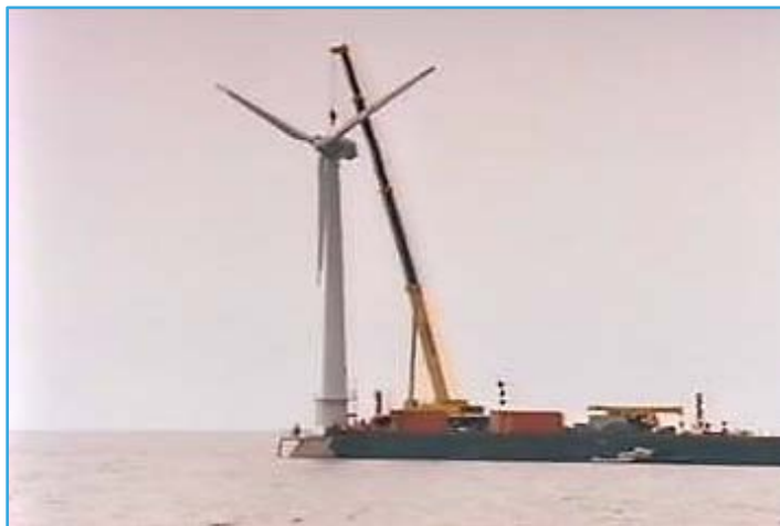
Figure 9-1. Removal of blades, Vindeby, Denmark
