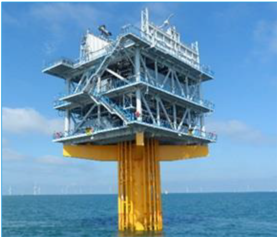
Figure 2-8. Offshore substation (London Array)
