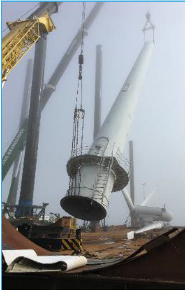
Figure 9-2. Removal of monopile, Vindeby, Denmark.
