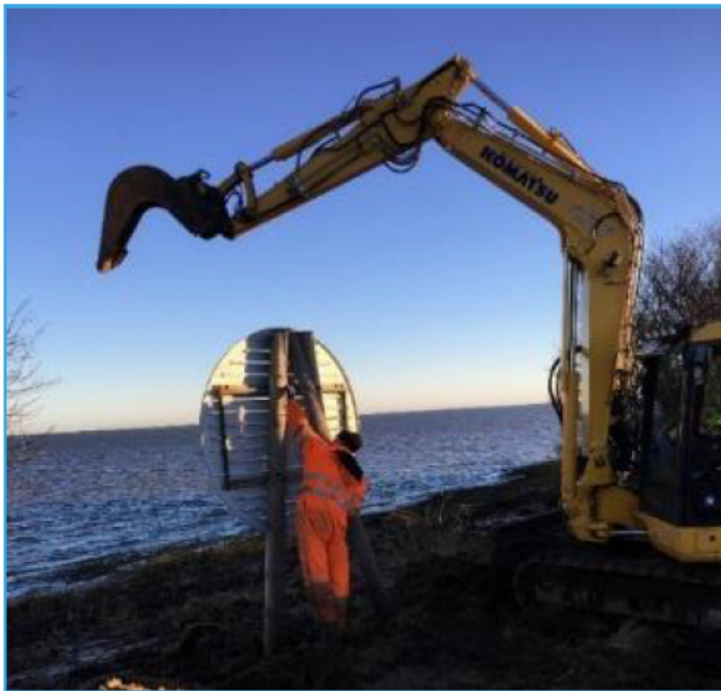
Figure 9-4. Dismantling of onshore substation, Vindeby, Denmark.
