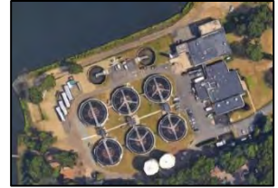
E – Central Swimming River Filter Plant
