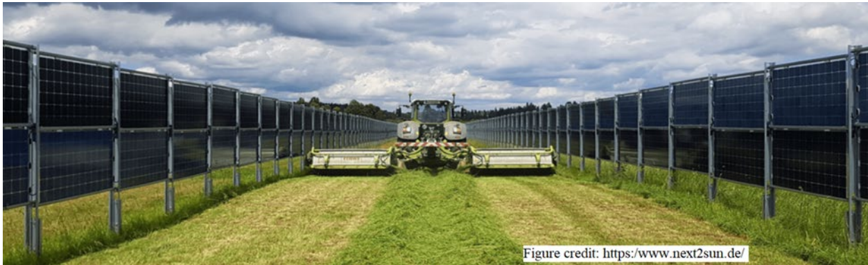
Figure C.3: A vertical bifacial array highlighting farm usage considerations. There is no limitation to the equipment headroom resulting in excellent ability to farm for all types of crops as well as grazing animals.
