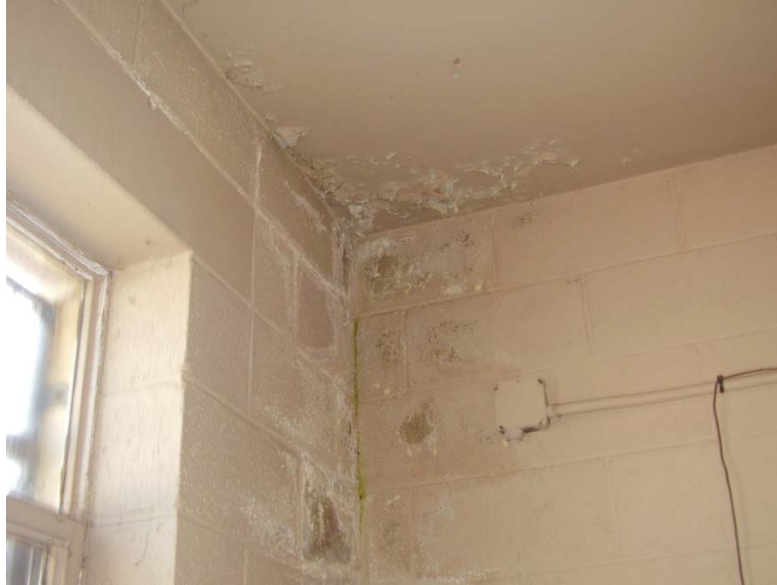
Water Damage inside Puchack Plant - Picture taken March 5, 2009.
