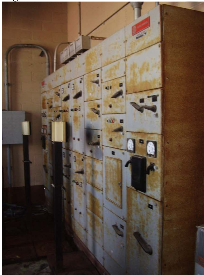
Electric Controls inside Puchack Plant - Picture taken March 5, 2009.
