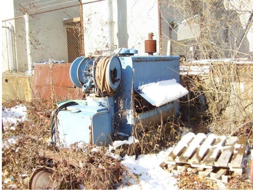
Davey Skid Mounted Air Compressor - Picture taken March 5, 2009, in the Puchack Plant Yard.
