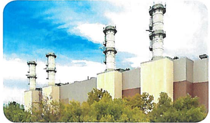
Design-Build procurement was utilized for Repowering We Energies Port Washington Combined Cycle Plant, where the Team acted as the Owner's Engineer.
