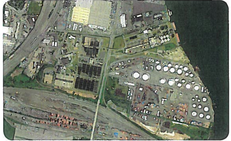
PVSC Plant Proximity to Newark Bay as a Flooding Source is driving the need for this Program.
