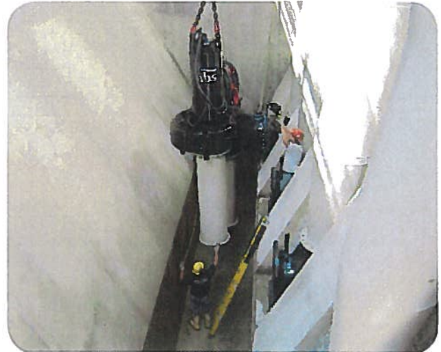
103 MGD CSO Pumping Station; Holyoke, MA. Utilized a "trench" wet well design to improve hydraulics for (4) 24,000 gpm pumps and to reduce accumulation of debris.
