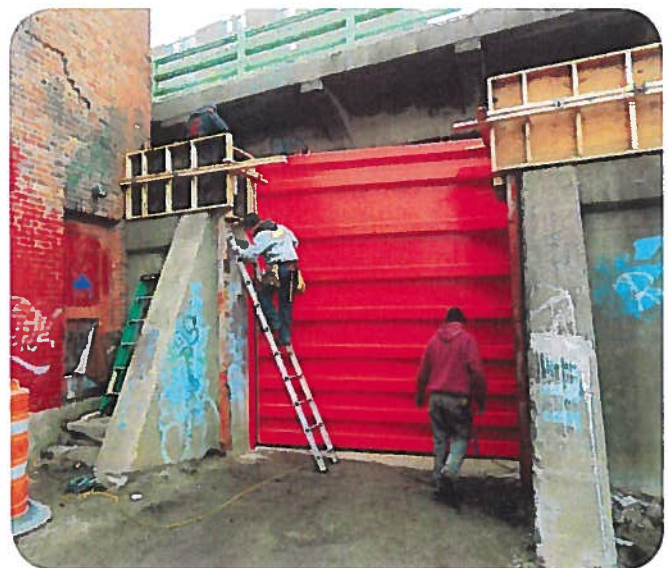
Gates similar to these designed by our Team in Haverhill, MA are required adjacent to the Sludge Storage Tanks.
