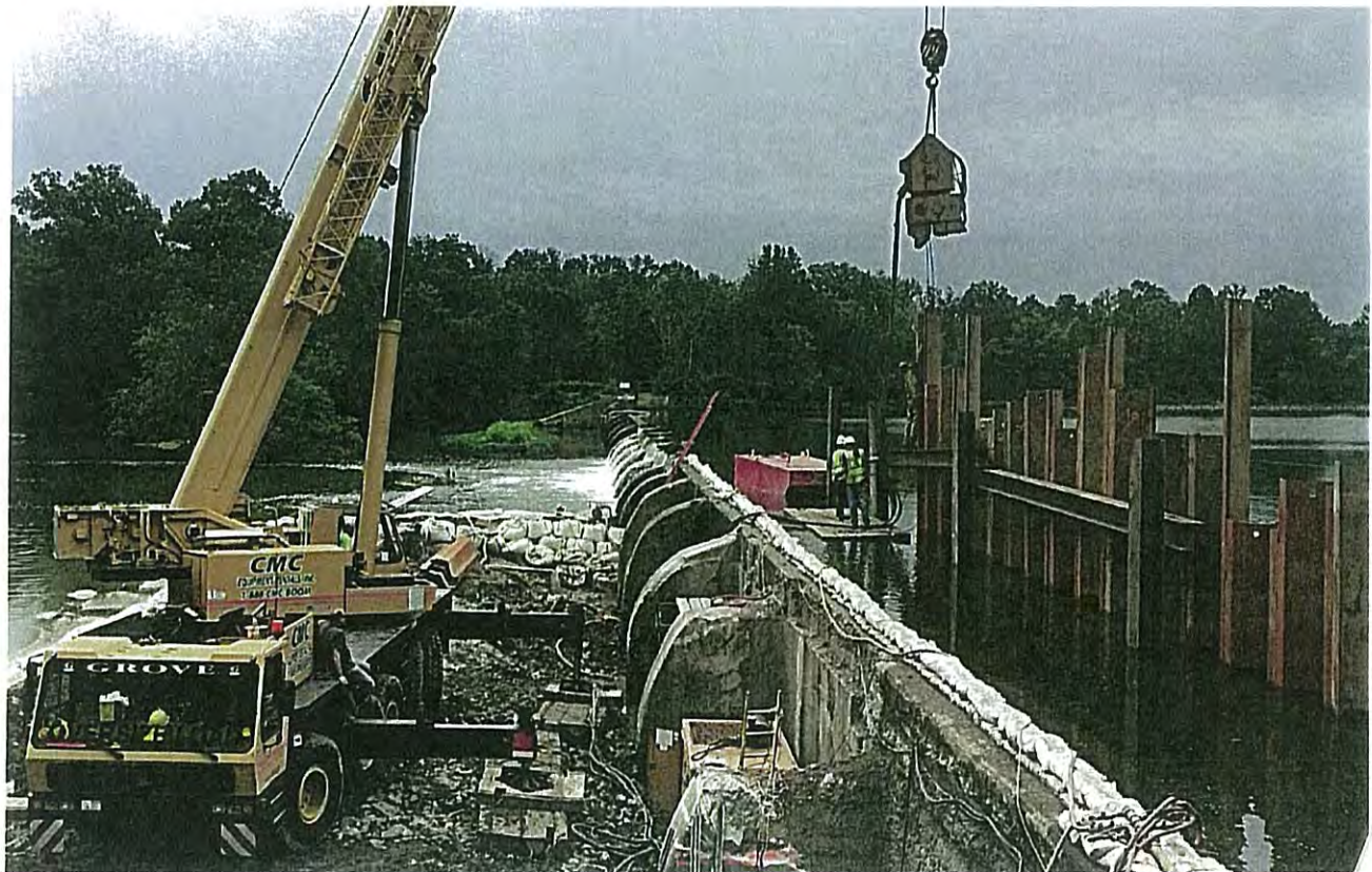
INSTALLATION OF STEEL SHEET PILE COFFERDAM
