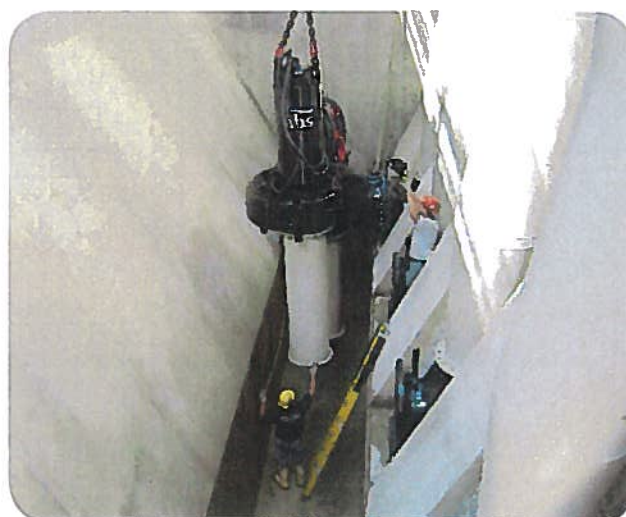
103 MGD CSO Pumping Station; Holyoke, MA. Utilized a "trench" wet well design to improve hydraulics for (4) 24,000 gpm pumps and to reduce accumulation of debris.
