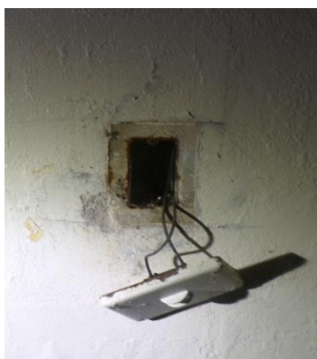
Figure 6 – Tampering of electrical outlets by incarcerated persons within cells in the RHU at Northern State Prison.
