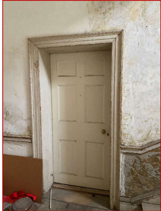
Door, Frame, and Hardware in Office No. 4
