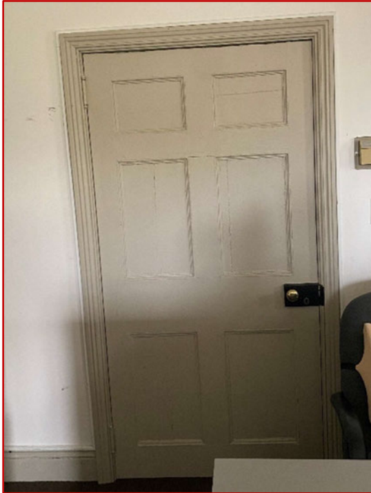
Door, Frame, and Hardware in Office No. 2
