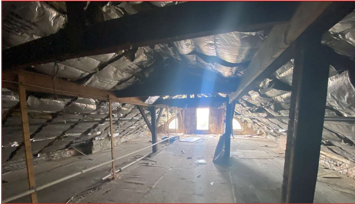
View of the Attic Space Viewing the South Interior Elevation
