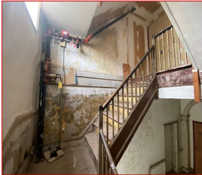
North Stairway Between Second and Third Floor
