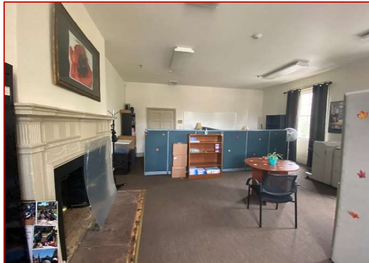
Second Floor North Wing Office No. 2 Looking at Historical Character Defining Feature No. 2 in Background
