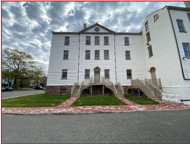
North Wing West Façade Exit Stair
