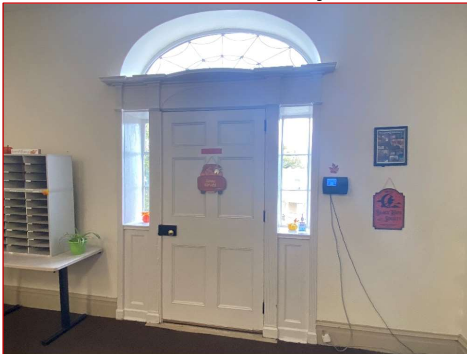
Door, Frame, Hardware, Sidelights, and Transom Above in Breakroom
