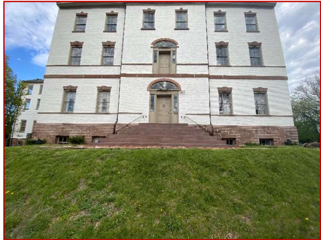
North Wing East Façade Exit Stair
