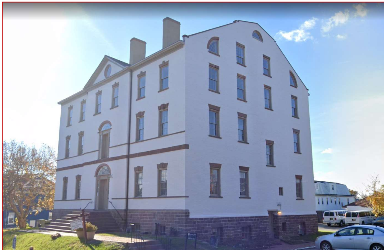
Northeast Corner of North Wing
