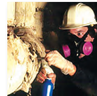
LEAD & ASBESTOS REMEDATION
