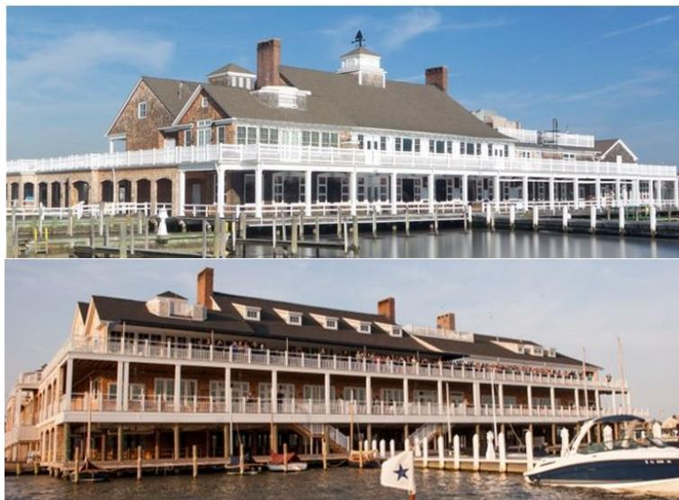
Figure 1: From Top: Before and After Elevation Pictures of Bay Head Yacht Club. During Superstorm Sandy, this historic structure had more than 3 feet of water on its first floor. With private funding, the Bay Head Yacht Club was elevated 8.5 feet. There was no change in the building footprint or the aerial coverage of the water as a result of the elevation.
