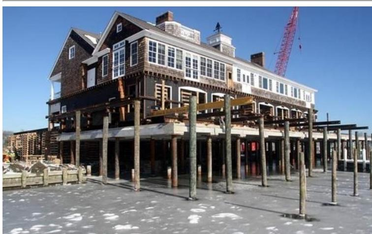
*Figure 2: This image was taken during the elevation of the Bay Head Yacht Club, an historic structure, after it was substantially damaged during Superstorm Sandy.*
