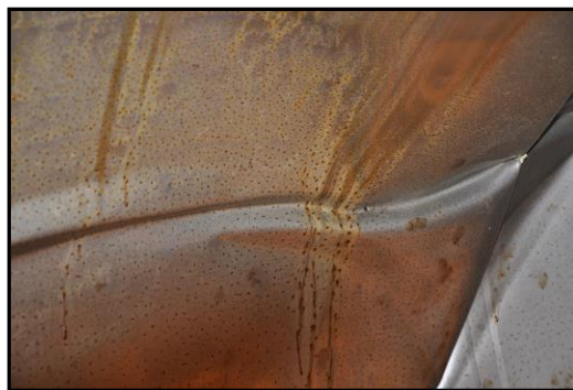
Figure 5 - Oily residues on interior walls of trailer
