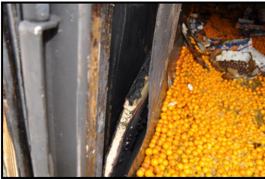
Figure 3 - Foam insulation in wall of trailer
